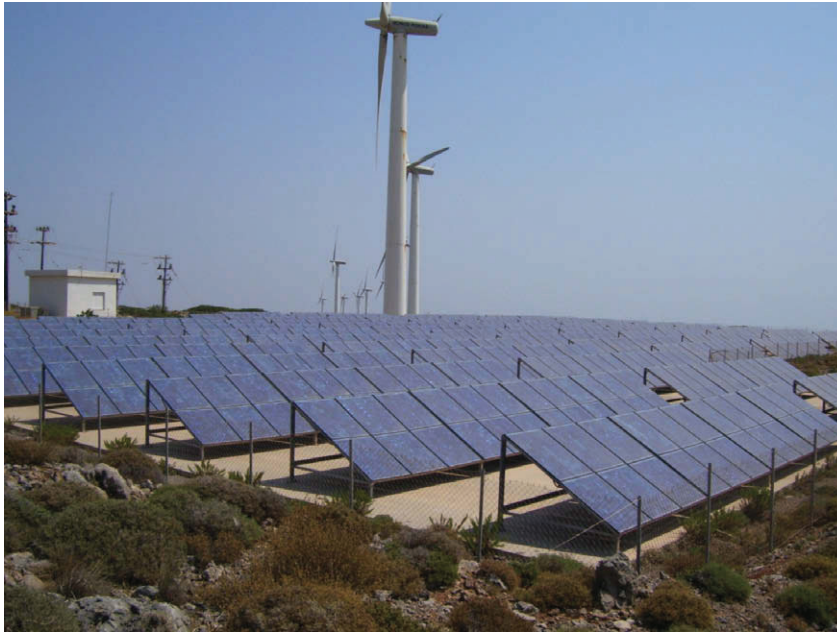
Fig. 1. View of the C. Rokas SA Photovoltaic Park. The PV modules are tilted at 30° and oriented south (the adjacent wind park in the background).
